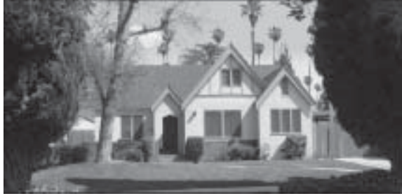
Figure 6 - Tudor Revival-style residence at 3669 Castle Reagh Place
