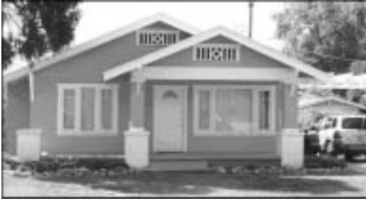
Figure 4 - Craftsman Bungalow at 4210 Highland Place
