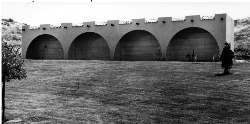
Olivewood's second mausoleum was a Spanish-style structure built in 1969 (and slightly modified since). (Olivewood Memorial Park)
