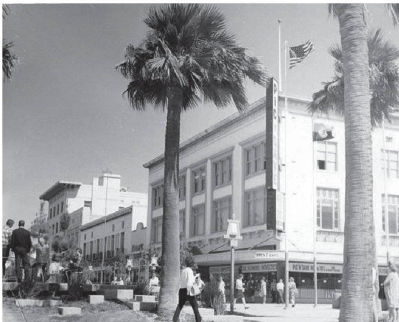
Riverside's Main Street Mall under construction in 1966 (City of Riverside Public Library)
